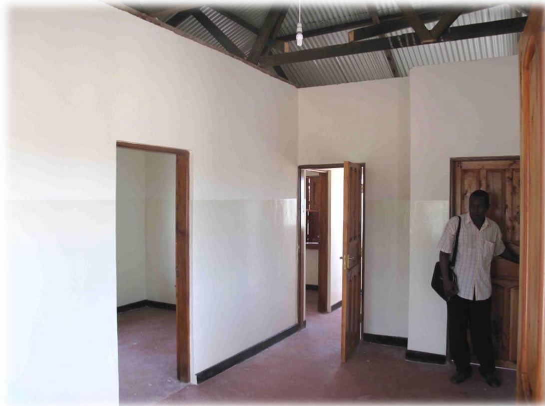
Garsen High School Bakery Project
